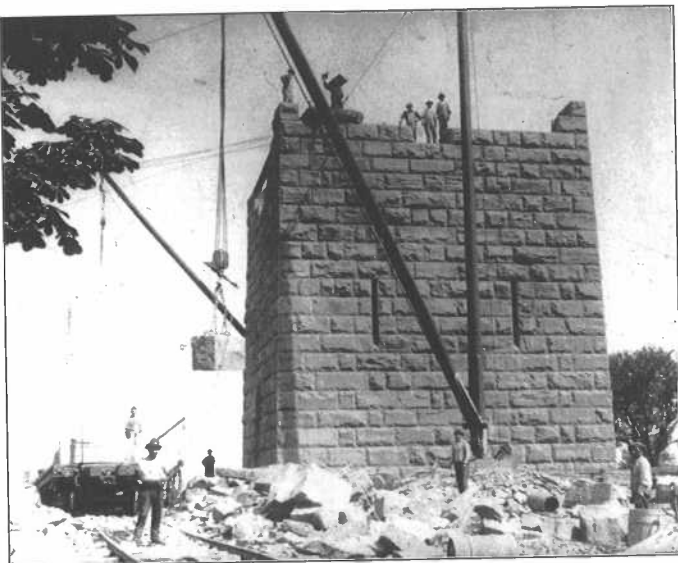
The monument under construction in June 1888. It was 40 feet tall at this point.
