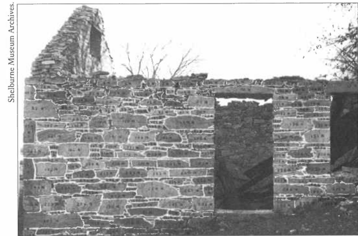
The Stone Cottage, with all its parts numbered, before it was taken apart and moved to Shelburne, 1949.
