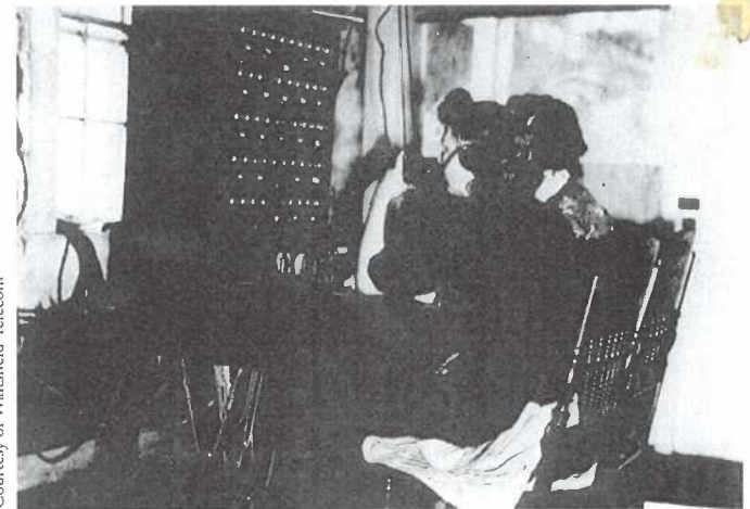
Elizabeth Long and Marguerite Moriarty answered calls on the switchboard at the old meat market in Waitsfield. Notice the wires coming through the window.
