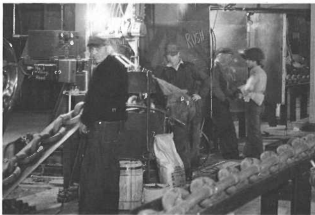
Welding anchor chain built for the U.S. Navy at Barre Products, Inc., a converted granite shed. Courtesy of Green Mountain Power Corporation.
