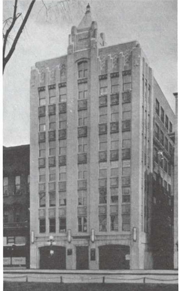
Service building, built in 1930 by architects Hutchins and French. Seven stories, 101 feet. Its fashionable Art Deco style has narrow shafts between the windows and an arrow design in the brick of the upper story. These decorations fool the eye and make the building seem taller than it is.
